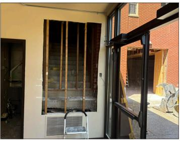
These are the original stairs that led up to the East Transept. They mirror the stairs on the West Transept (8th Street entrance). These were walled in when the present elevator and stairs were erected.
