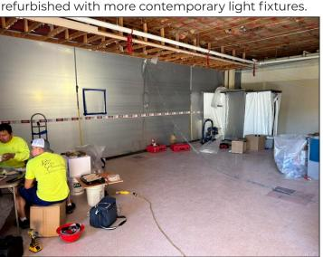
Plastic barriers confine the asbestos abatement being done in the kitchen and "Front Section" of the parish hall. The abatement workers put on hazmat suites and enter the abatement area through the tunnel on the far right.
